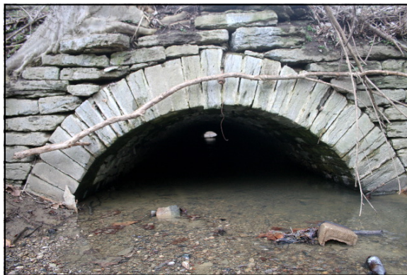
One of two 8-foot x 4-foot stone arch canal culverts built by David Guard in canal sections 6 and 7 along Oberding Road. Photo by Kim Ziegel
